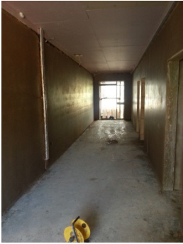
Ground Floor Corridor
