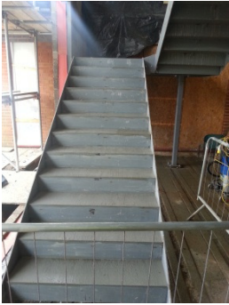
New stairs treads concreted
